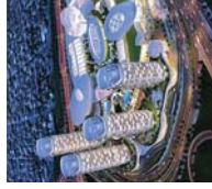
Location: Turkey (Istanbul) Project: Mall of Istanbul
